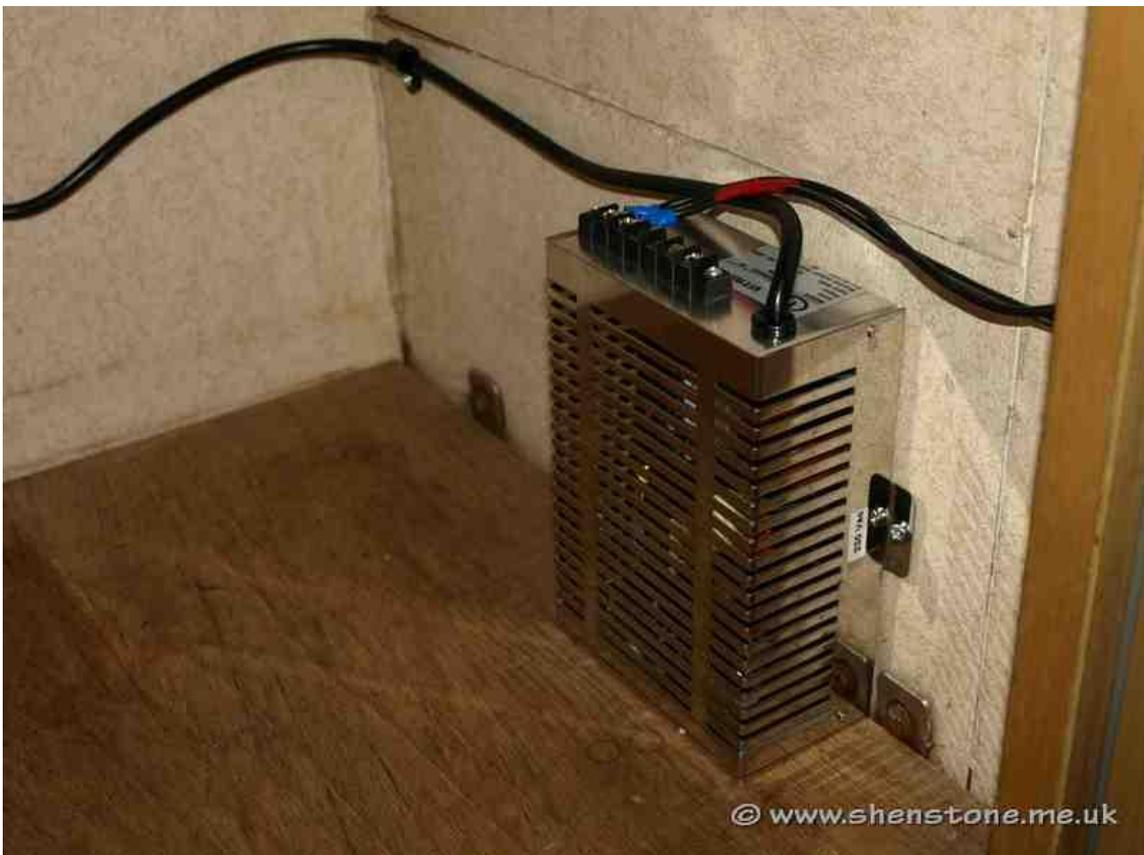
Finally, being a yorkshireman and tight with money, and because of the position inside a cupboard, instead of purchasing some expensive kit to fasten it in I used a couple of brackets fastened into the lower door fittings which were unused from another project
