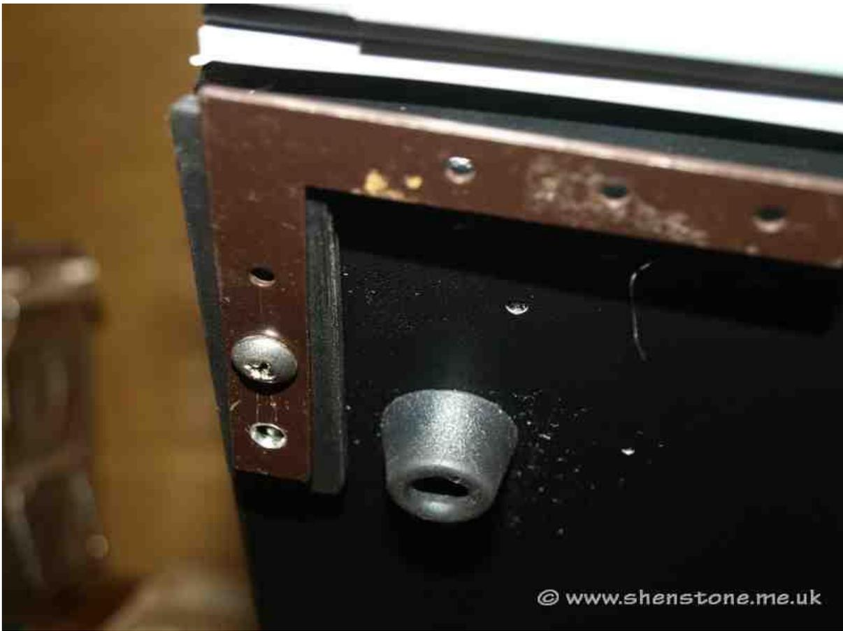
And added another couple of brackets fastened to a screw in the frame on the top of the fridge to ensure that it is 100% firm in place
