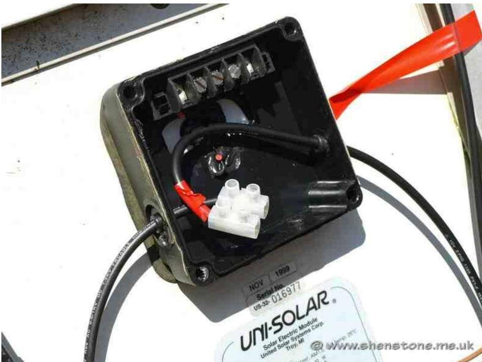
But for "belt and braces" the whole connection box was sealed with flexible sealant as well
