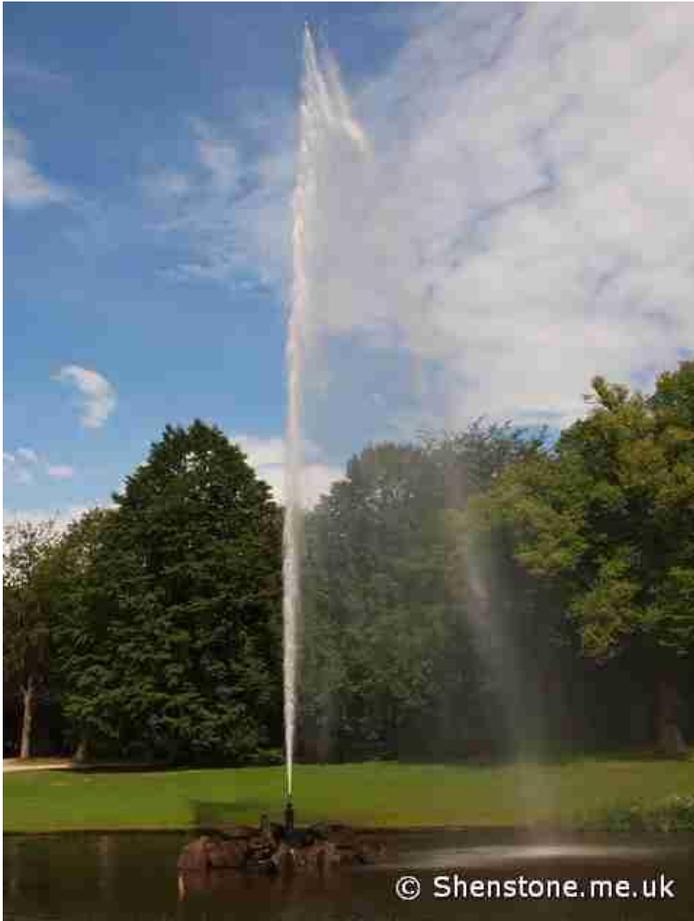
The fountain is powered by the pressure of the water dropping 122 meters, through a 40 centimeter iron pipe made from a man-made lake. The fountain can reach a height of 90 meters although it is usually to half that height to conserve water (as in the picture)
