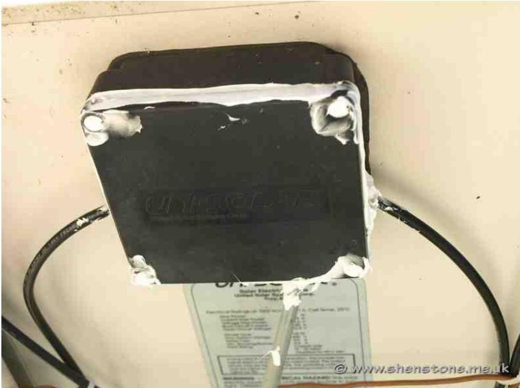
I would have liked to have virtually no loose wires, but that would have meant cutting the connections off the solar panel so I arranged them on the rear. it will mean there is spare cable if I need to adjust things so maybe not a bad thing
