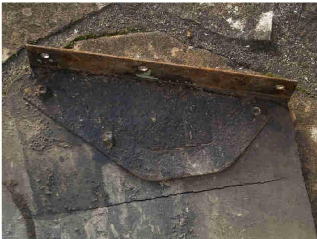
To complete this work 22 nuts & bolts or rivets had to be addressed. 20 of them ended up being cut off.
